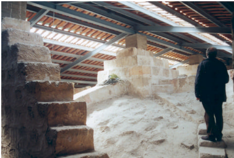
Figure 11: Masonry dead weights placed on top of the arches and vaults of the nave
