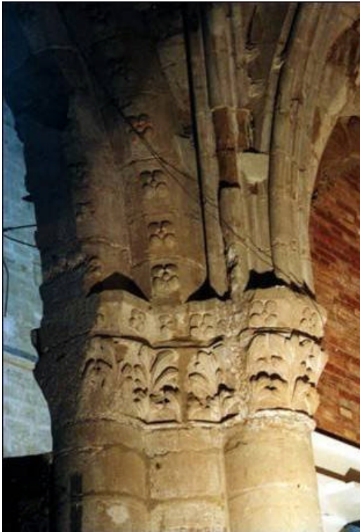
Figure 5: Tarazona Cathedral. Lesions related to excessive compression at the springings of the aisle arches.
